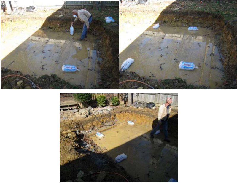
Figure 7. Ice Bag Positioning in Excavation
