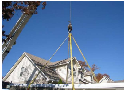
Figure 7. Ice Bag Positioning in Excavation
