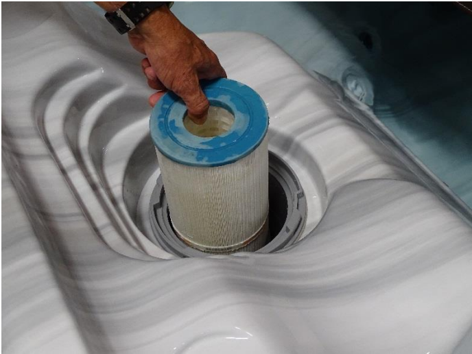
Figure 16. Drop in filter removal
