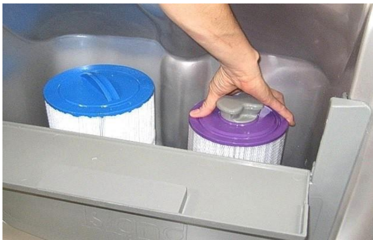
Figure 18. Screw-in Filter Removal
