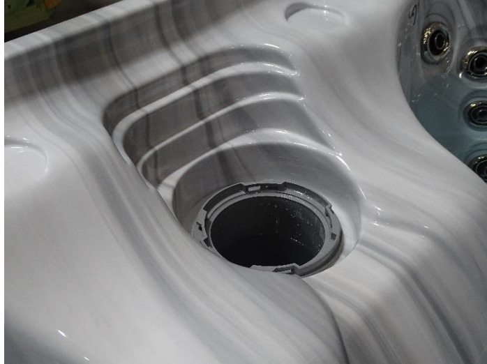
Figure 17. Empty filter housing
